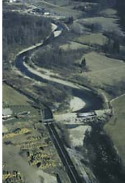
Titan mill stream along the Kamniška Bistrica River.
